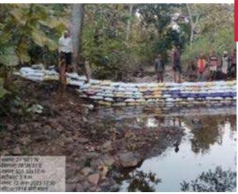
Picture 10: Construction of Check Dam under Wildlife Conservation in Chhindwara Project Division of MPRVVN.
