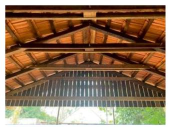
**Figure 4.** DIS Anganvadi with Glulam coco palm sections.
