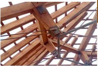
**Figure 3**. Detail compression posts with steel rod tensioning with Glulam coco palm timber.
