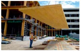
Figure 5. CLT used as floor, wall and structural panel.
