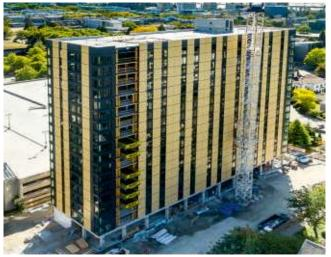
Figure 4. Mass timber construction using CLT and GLT.
