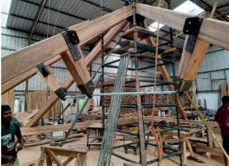
**Figure 2.** Full scale erection of pyramid roof in coco palm glulam at the workshop.
