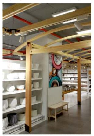
Glue laminated columns and Beams
