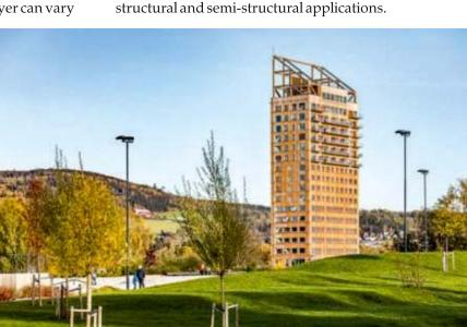
Figure 3. Tallest timber-based structure in the world at 85.4 m, the Mjostarnet building in Norway (courtesy: Voll Arkitekter).
