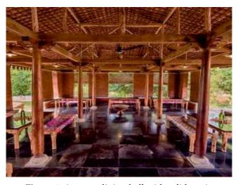
**Figure 5.** A resort dining hall with solid section short span coco palm timber.
