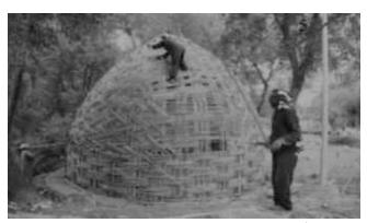
**Figure 1.4:** Erection of domed roof
