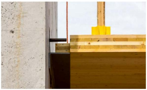
Figure 8. Column to CLT Slab connection, UBC (Photo courtesy: KK law [6]).
