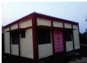
Fig. 2: A model 2-BHK bamboo reinforced concrete house constructed in school premise near IIT in 2014 (Sponsoring agency BMTPC)
