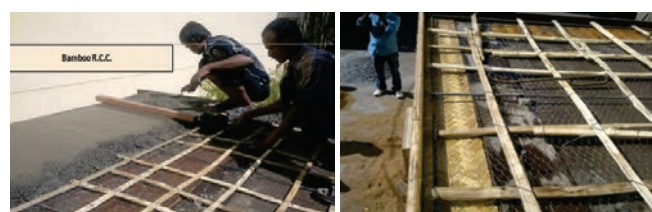
Construction at IPIRTI, Bangalore with Bamboo reinforcement
