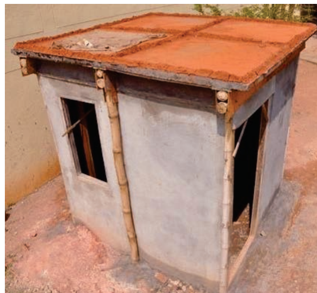
Fig. 2: A model 2-BHK bamboo reinforced concrete house constructed in school premise near IIT in 2014 (Sponsoring agency BMTPC)
