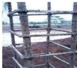
Fig. 1: Chemically treated bamboo reinforced bar used in column
