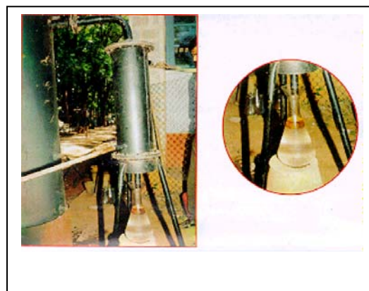
Close up of Condenser and receiver
